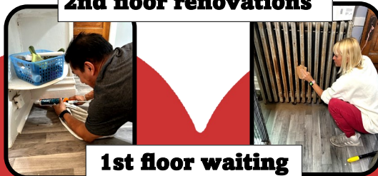
2nd floor renovations
